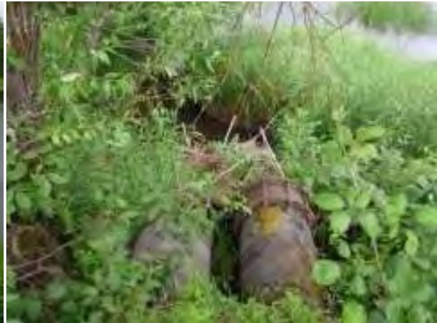
Photo 20. Pipes draining Wetland B through the levee into Wetland B, 5-29-13.
